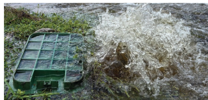
Storm Water & Hydrovac
